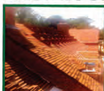
Handmade clay tiles roof in progress
