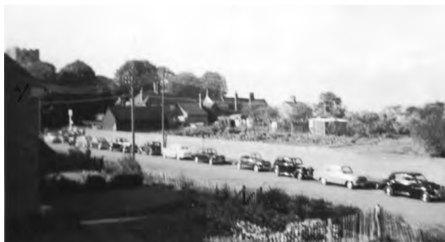
View from Chiltern Avenue, Church on left, probably early 1950s
