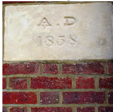
Flemish Bond - Methodist Chapel - High Street
