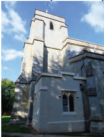
The Eaton Bray Church toilet by John Hockey
