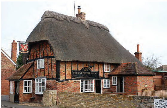
The Carpenters Arms, Slapton
