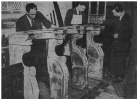
Restoring the Miserere seats in the chancel
